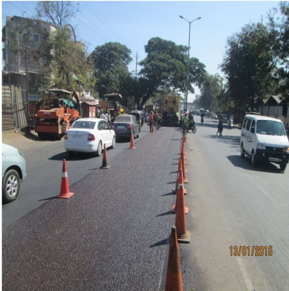
Microsurfacing Laying
